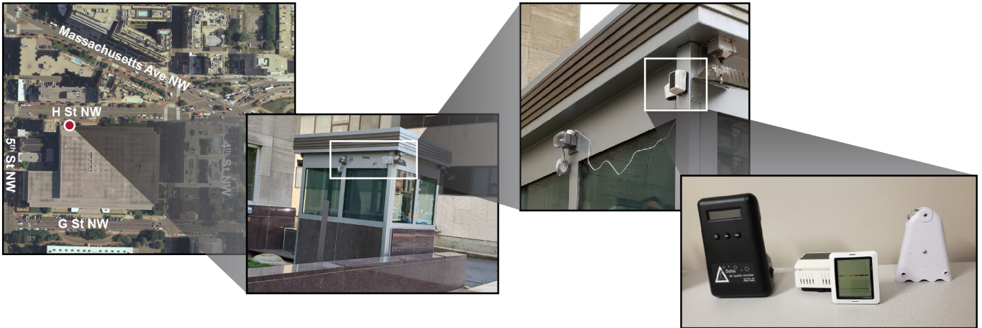
Figure 9: Low-Cost Sensors Deployed on the GAO Building
