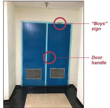
Restroom sign located too high, located on the door, and lacks raised characters or braille. Door hardware also requires pinching or grasping to open.
