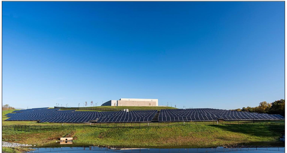
Figure 9: Social Security Administration, National Support Center - On-site Solar Panel Array outside the Data Center
