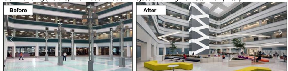
GSA Building (Before) and Modernization Project Showing New Stairwell (After)
