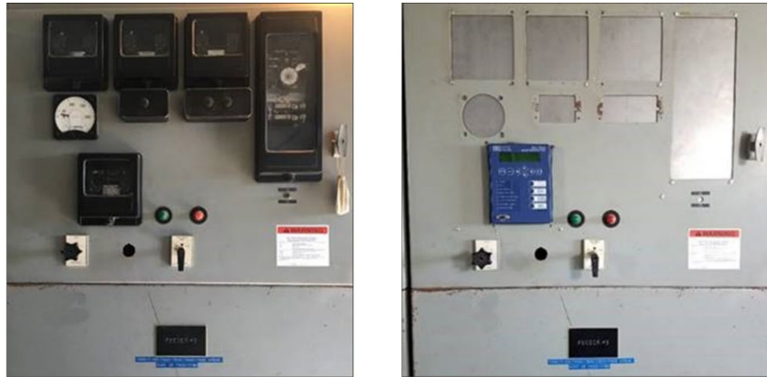
Figure 2: Electrical Panel on a Military Installation before (left) and after (right) the Utility System was Privatized
