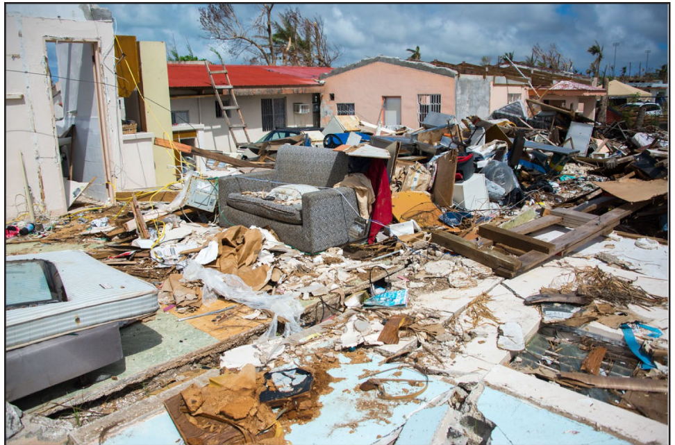
Figure 2: Damage Caused by Super Typhoon Yutu
