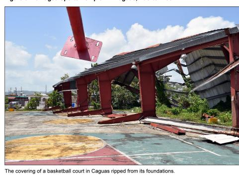
Figure 6: Damaged Sports Complex in Caguas, Puerto Rico
