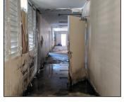
Interior damages to a school in Puerto Rico from water infiltration with standing water and molded walls.
