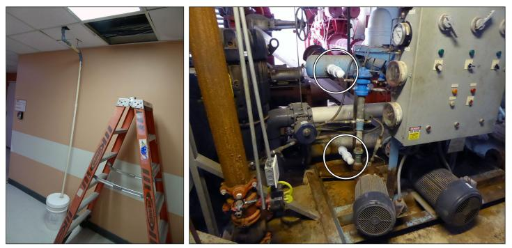
An example of a temporary measure to capture continued water infiltration from the facility's damaged roof.
