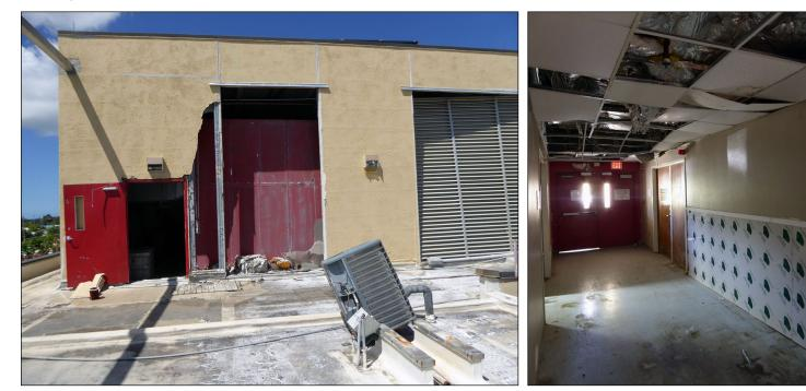
A section of the facility that was sheared off during the hurricane leaving the building's ventilation units susceptible to outdoor conditions. Source: GAO. | GAO-20-54
