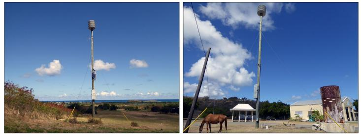
Two tsunami warning system stations in St. Croix, U.S. Virgin Islands. Each station comprises a pole, a siren head to broadcast warnings, a solar panel, stabilizing guy wires, and other ancillary equipment.
