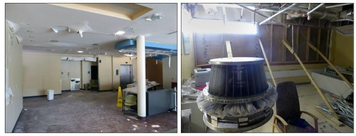
Damage to the hospital's roof allowed water to infiltrate the facility, severely damaging check-in areas, hospital rooms, medical equipment and records, and offices.
