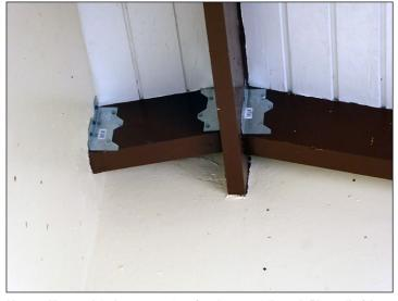
Home with completed permanent roof replacement through Phase II of the STEP pilot program, which included the installation of hurricane clips to increase the roof's resilience during hurricane-strength winds.
