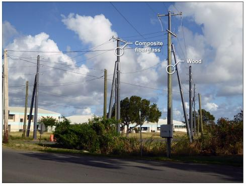
Damaged wooden utility poles for electricity distribution are being replaced by composite fiberglass poles that can withstand 200 mile per hour winds.
