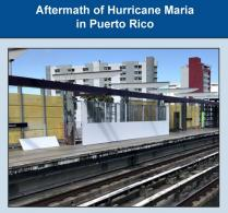
A white wall temporarily replaces the yellow wind and safety screen that was damaged by hurricaneforce winds at an elevated station platform of Tren Urbano, San Juan's rail transit service.
