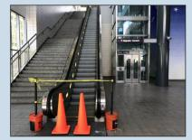
Out of service escalator at Tren Urbano station, which sustained damage to electrical parts due to water intrusion from the hurricane.
