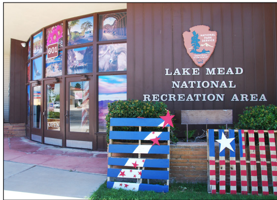
One-way vinyl window film with nature photographs provides security for the front desk attendant at a National Park Service field unit.
