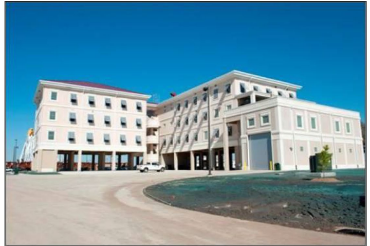
Station Sabine Pass rebuilt to withstand 100 year flood, category III hurricane wind speeds.
