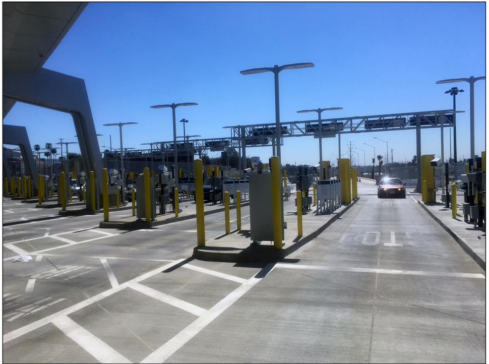
Figure 11: License Plate Readers and Radiation Portal Monitors on the Southern Border
