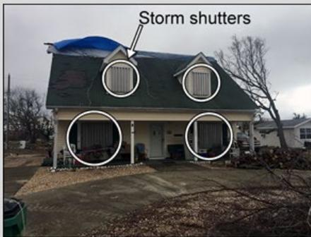
Some examples of hazard mitigation measures are house elevation, metal roofs, and storm shutters.
