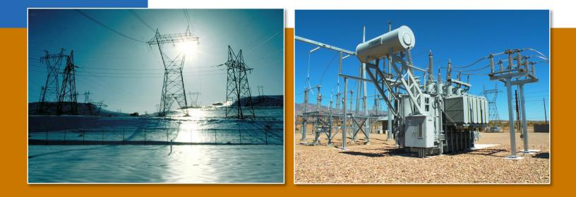
The cover images depict electric power transmission equipment that can be affected by geomagnetic disturbances. On the left is a photograph of electric power transmission lines, in which geomagnetic disturbances can create geomagnetically induced currents. On the right is a photograph of a transformer, which can become the source of virtually all geomagnetic disturbance-induced issues on the electric power grid.
