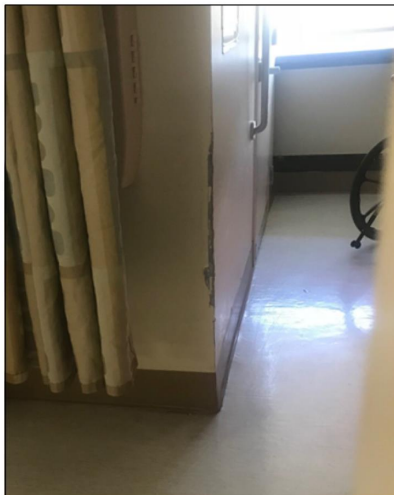
Wall corner with damaged plaster and paint
