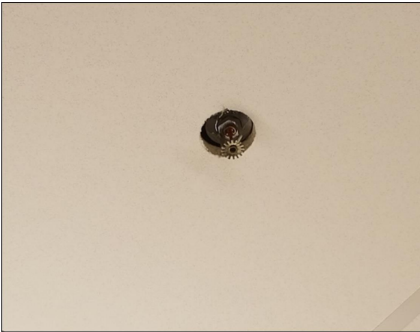
Fire sprinkler head missing metal plate
