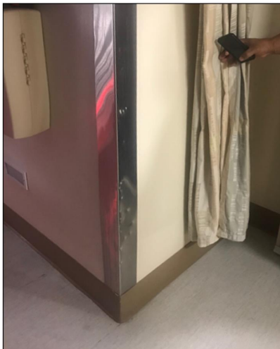
Wall corner with metal protective cover
