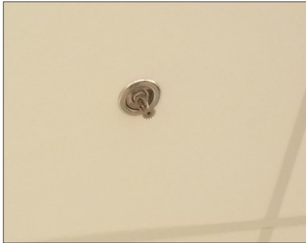
Fire sprinkler head with proper configuration
