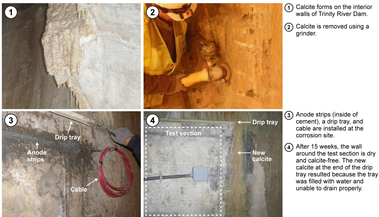
Figure 3: Use of Electro-Osmotic Pulse Technology by the Department of Interior's Bureau of Reclamation to Prevent Water Leaks on the Trinity River Dam, 2011
