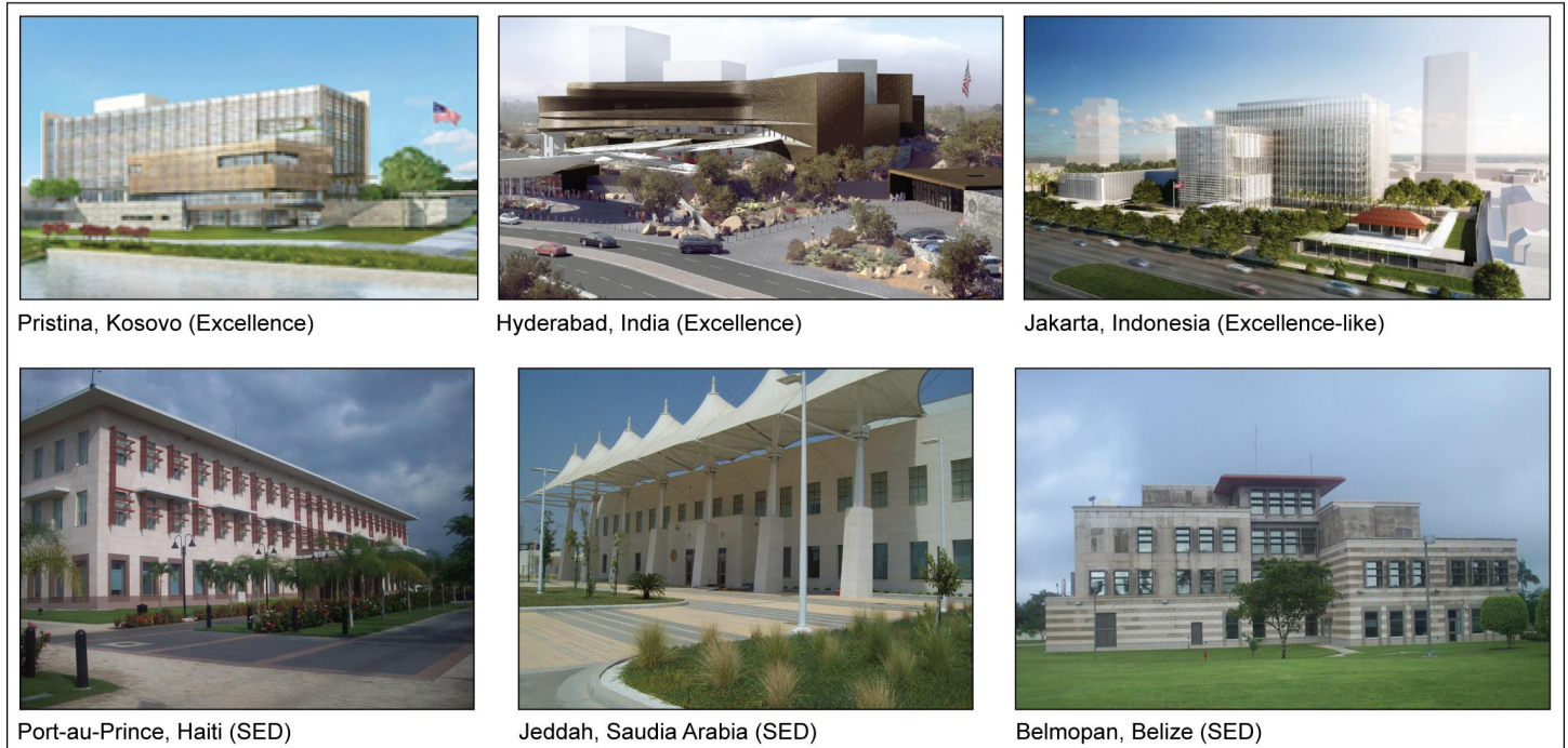
Figure 9: Examples of More Customized Exterior Designs (top row) Compared with More Standardized Exteriors of Some Standard Embassy Design (SED) Projects (bottom row)
