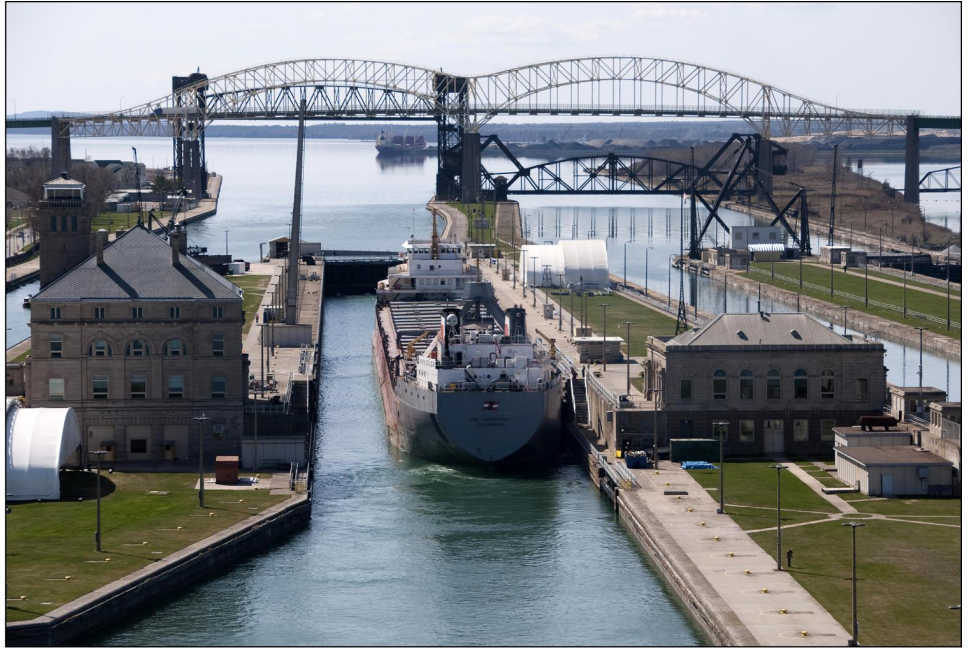
Figure 6: The Poe Lock, Located at Sault Ste. Marie, Michigan, and Managed by the U.S. Army Corps of Engineers
