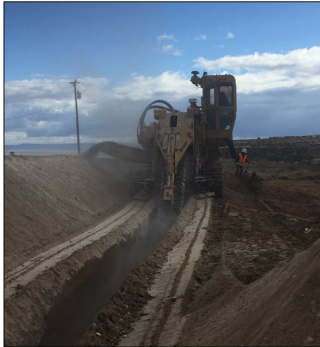
Digging a trench for sewer pipes.
