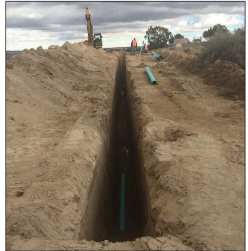
Laying sewer pipes.
