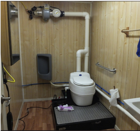
Bathroom with separating toilet and sink.
