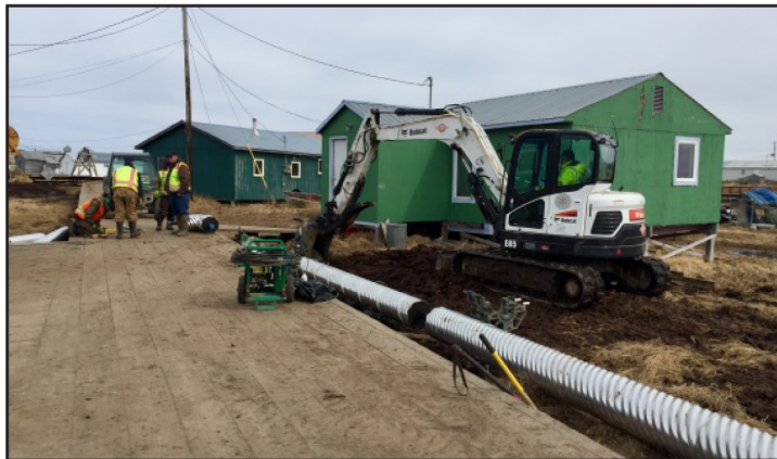
Figure 1: Water Infrastructure Project in Eek, Alaska (April 2017)
