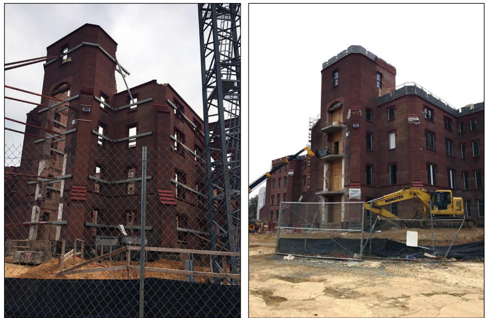
Figure 2: The Center Building at St. Elizabeths in 2016 (left) and 2018 (right)
