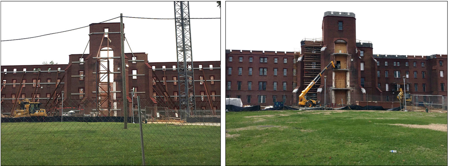
Figure 1: The Center Building at St. Elizabeths in 2016 (left) and 2018 (right)
