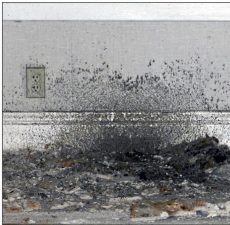
Portions of the ceiling have collapsed, spraying debris on to the floors and walls.
