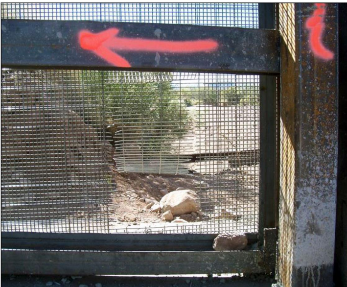
Breach in modern mesh pedestrian fencing
