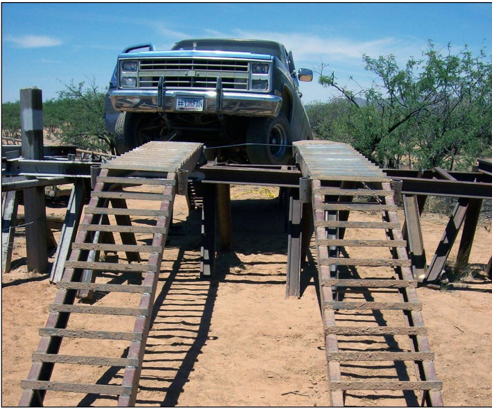
Truck attempting to defeat vehicle fencing with ramps
