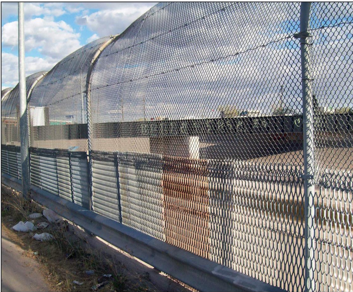
Legacy expanded metal style pedestrian fence
