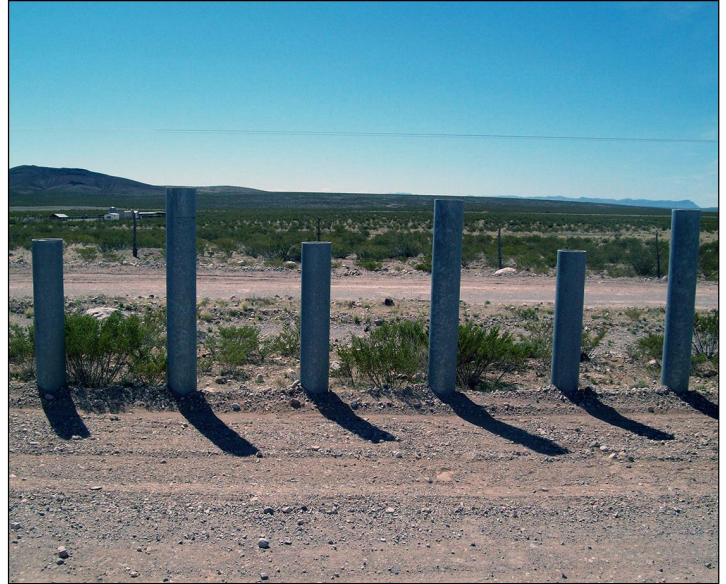
Modern bollard style vehicle fencing
