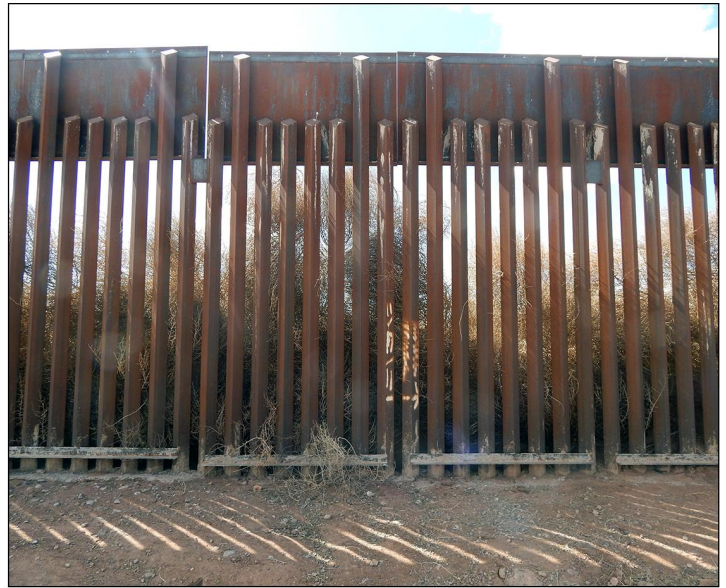
Modern bollard style pedestrian fence
