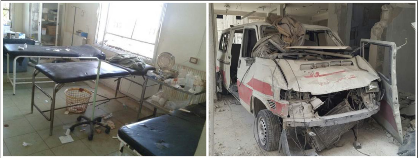
Figure 1: Damage to Health Facilities in Syria after Aerial Attack, Tel Shehab, Dara'a Province (left) and Al Khaf, Rural Damascus (right)
