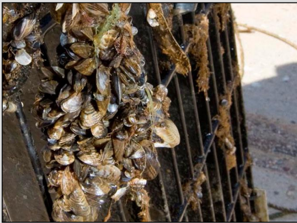
Source: Bureau of Reclamation. | GAO-16-49 Quagga Mussels covering infrastructure
