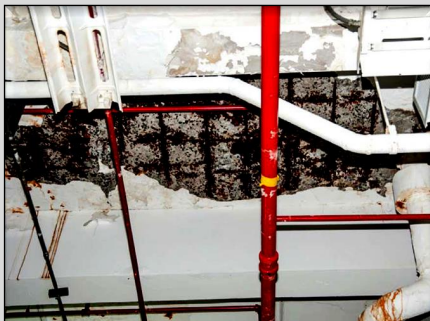
Source: Y-12 National Security Complex. | GAO-15-499
