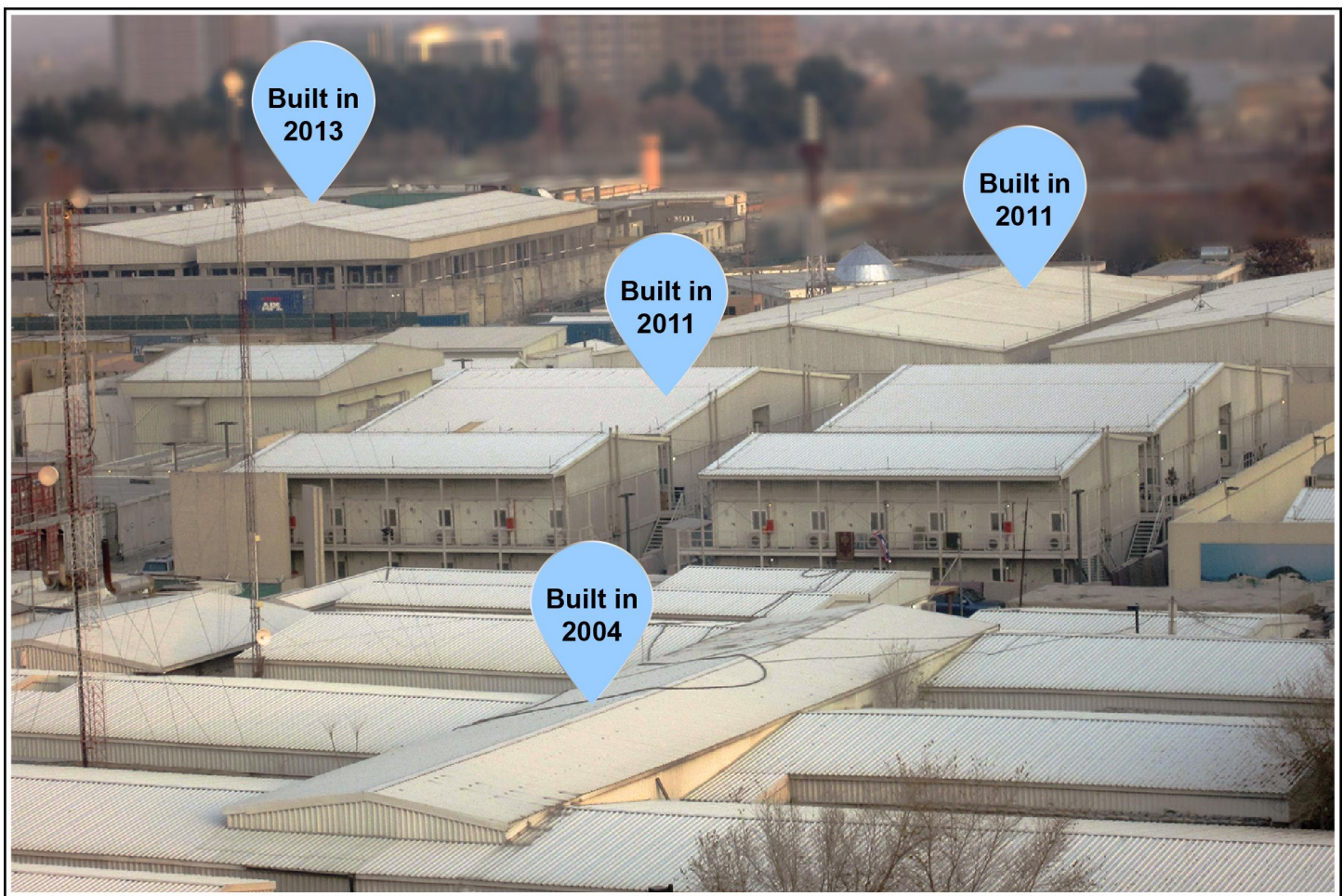
Figure 3: U.S. Embassy Kabul, Temporary Facilities
