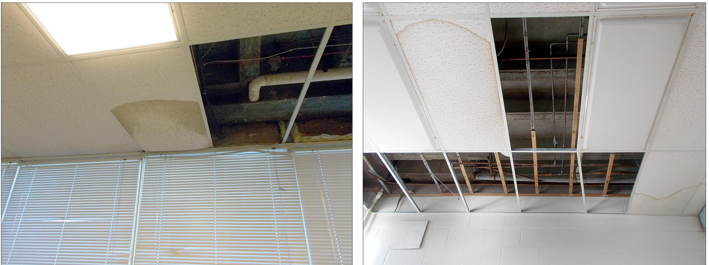
Figure 5: Damaged or Removed Classroom Ceiling Tiles Due to Leaks in Recently-Installed Roofs
