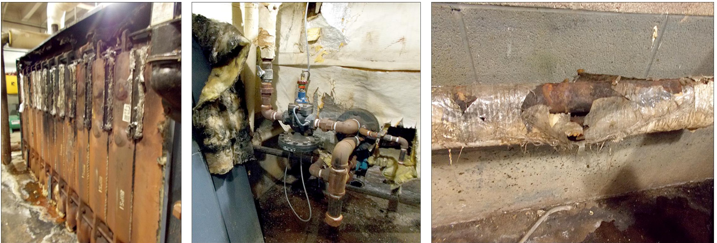
Figure 3: Aging Boiler Systems at a Bureau of Indian Affairs-Operated School Built in 1959
