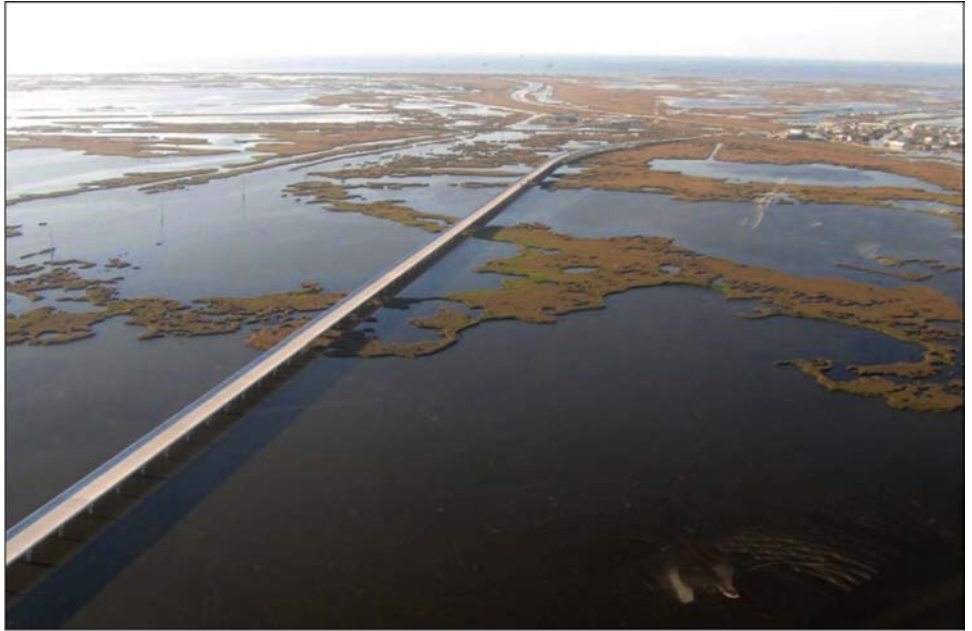
Figure 1: Louisiana State Highway 1 Leading to Port Fourchon
