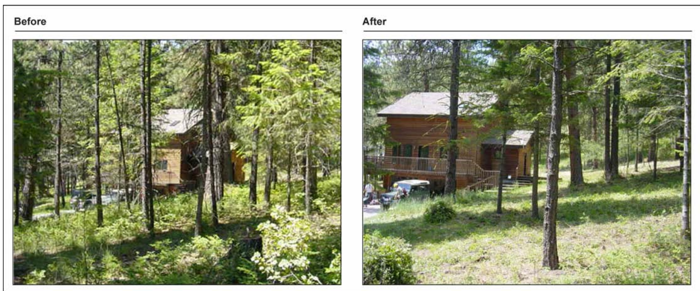
Figure 2: A Private Home in Montana Before and After Wildland Fire Mitigation Work Was Completed Using Title III Funds
