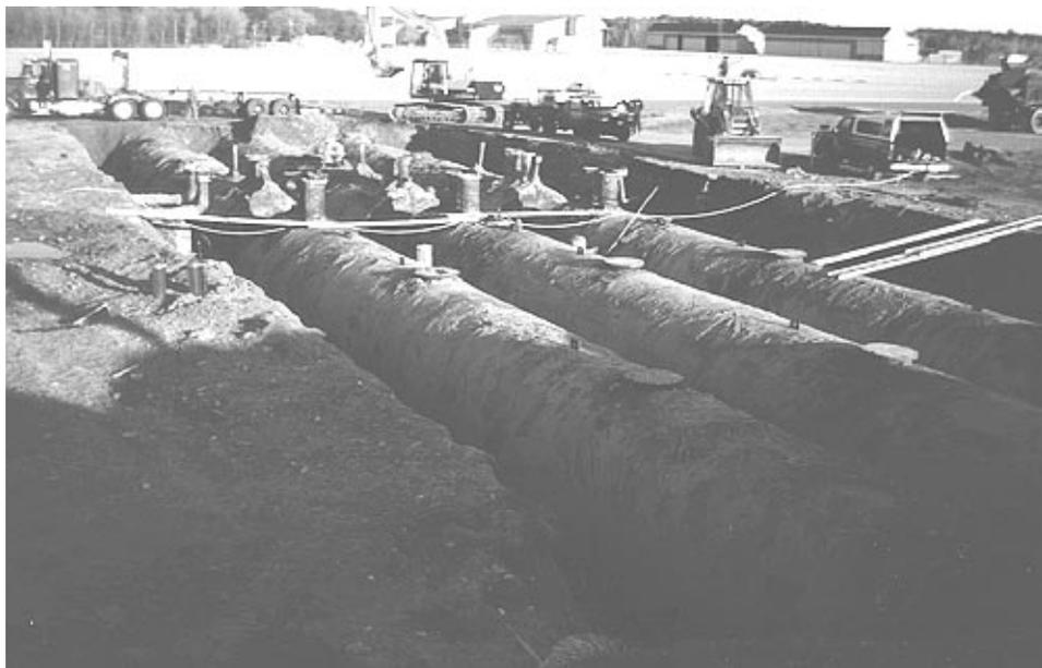
**Figure 4: Underground Fuel Storage Tank Removal at Pease Air Force Base**
