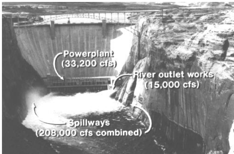
Figure 1.1: Water Release Capacities of the Glen Canyon Dam's Powerplant, Outlet Works, and Spillways
