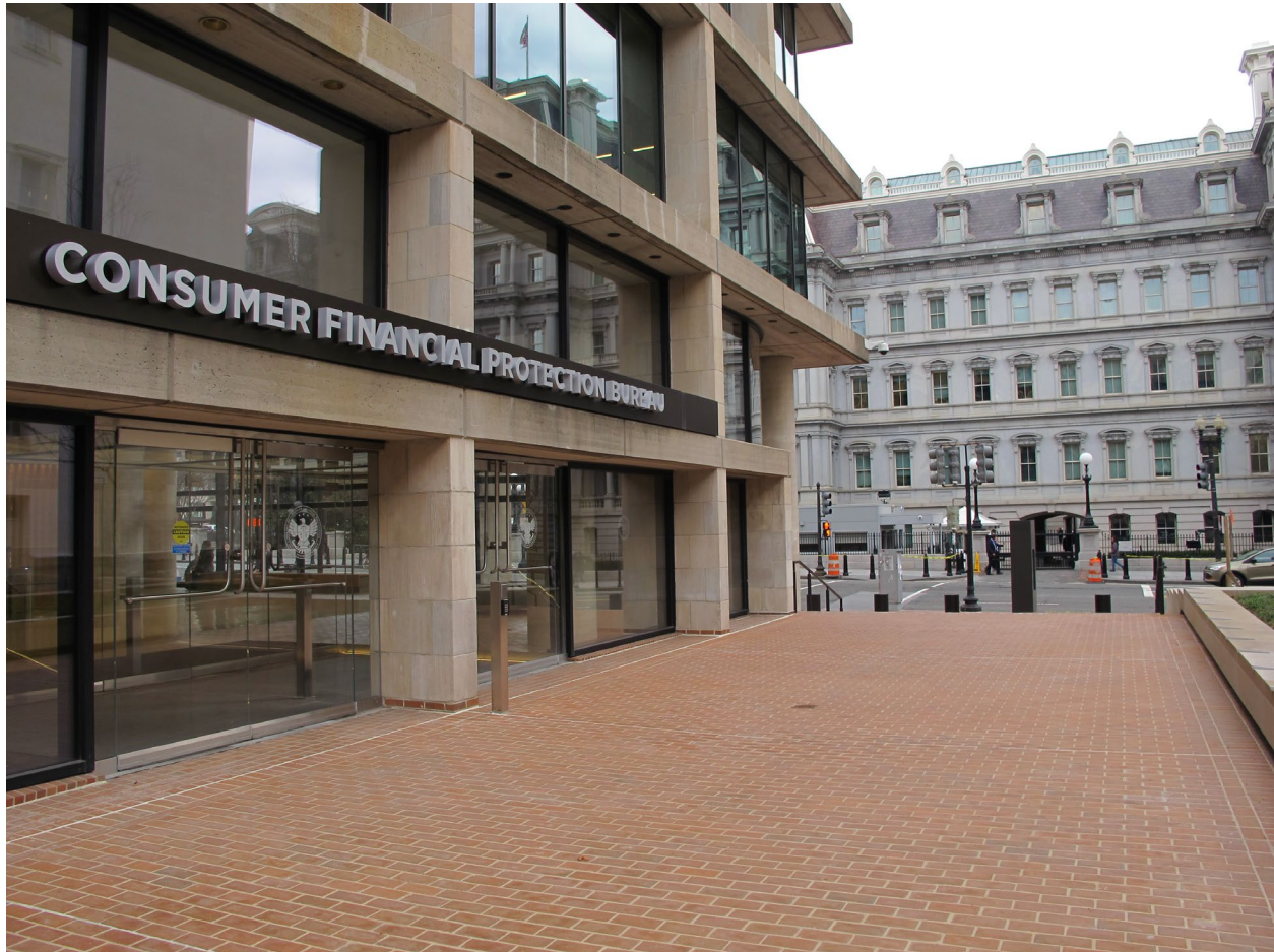
Image 1: Washington D.C Headquarters Building
