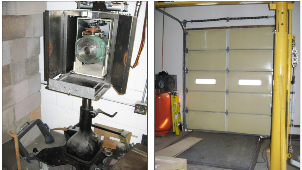
Figure 7: Irradiator on Wheels and Loading Dock
