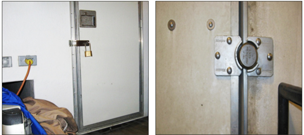
Figure 4: Standard Padlock for Darkroom Door and High-Security Lock for Door
