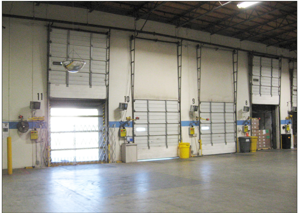
Figure 10: Loading Dock with Roll up Doors
