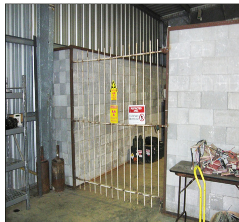
Figure 6: Open Rolltop Door and Barrier Not Extending to Ceiling
