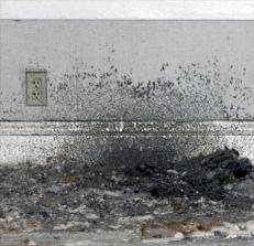
Portions of the ceiling have collapsed, spraying debris on to the floors and walls.
