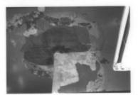
Major Ceiling Damage From Leaking Roof Causing Crumbling Plaster in Classroom
