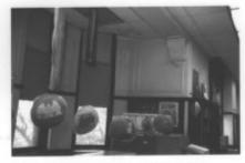
Library Ceiling Damage Caused by Leaking Roof
