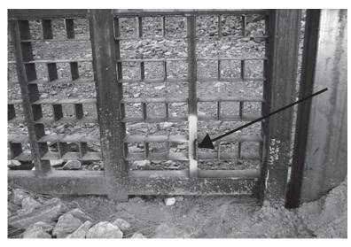
Figure 6: Examples of Repaired Breaches in Newer Fencing
