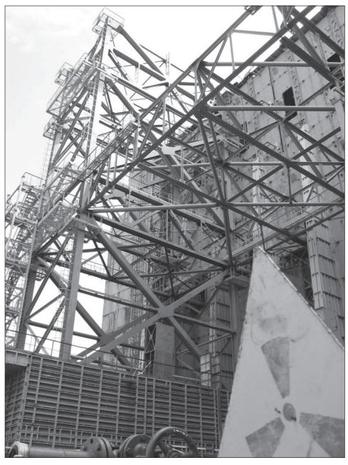
Figure 4: Stabilization Work for the Western Wall
