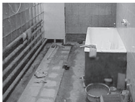
Source: DOD. Before renovation
