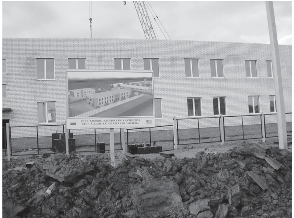
Figure 3: Administration/Cafeteria Building under Construction, November 2005
