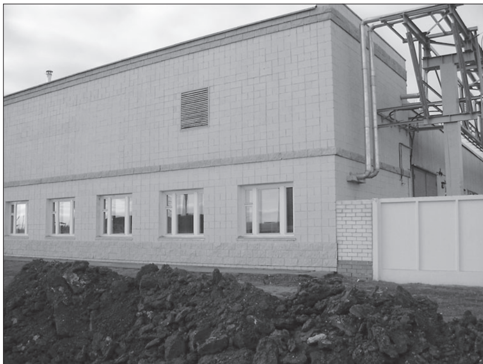
Figure 2: Completed Firehouse at Shchuch'ye, November 2005
