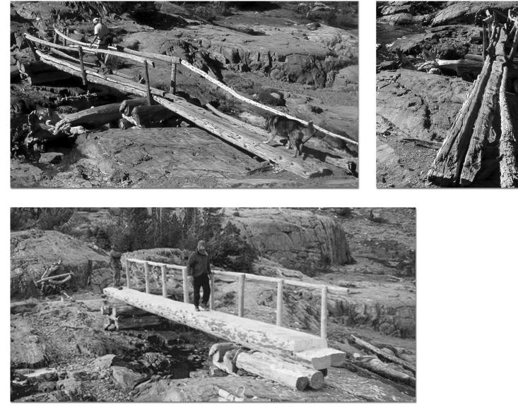
Figure 2: Funding Transfers Delayed Replacement of a Failing Backcountry Bridge (Inyo National Forest, California)
