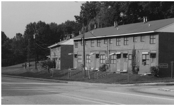
Tobe Hartwell Courts prior to demolition.
