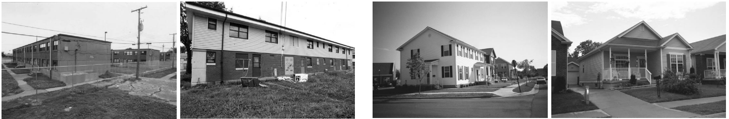
Cotter and Lang Homes prior to demolition.
