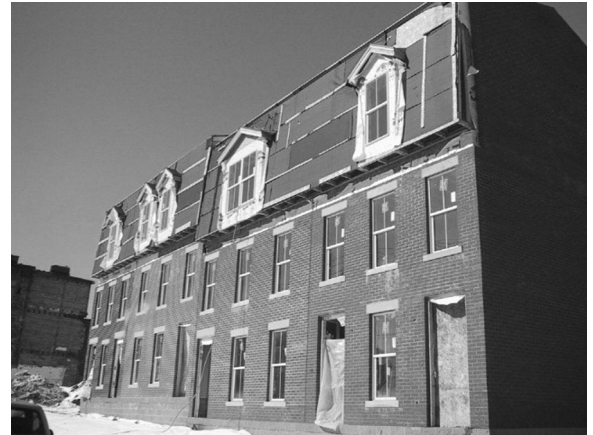
Off-site construction under way.
