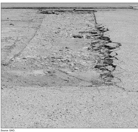
Figure 7: Crumbling Concrete Outside Cargo Center at Whiteman Air Force Base, Missouri
