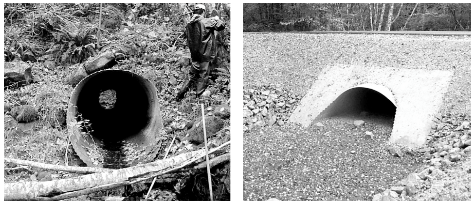
Figure 1: Culvert Before and After Replacement
