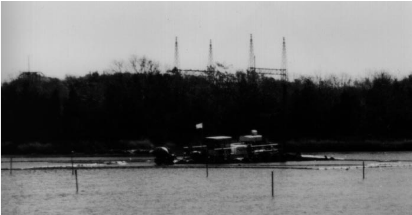
Figure I.3: Dredging Facility at New Bedford Hot Spot
