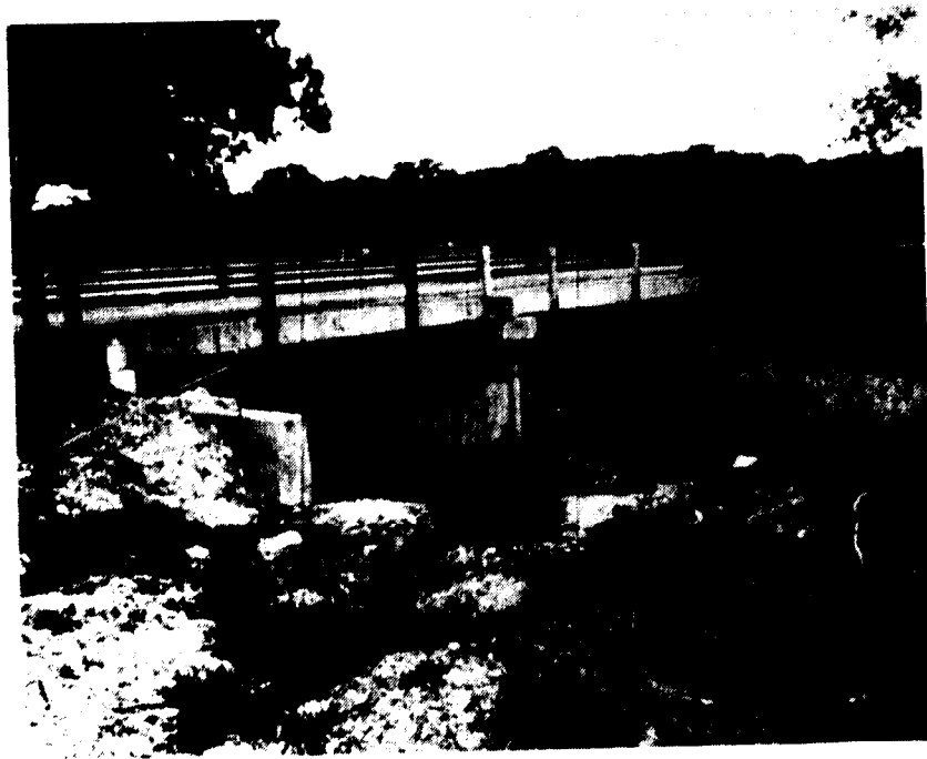
Top And Side View Of A Bridge Built By Washington County, Arkansas' Employees With Their Own Pre-cast Concrete Sections. The Cost Was Less Than $20,000.
