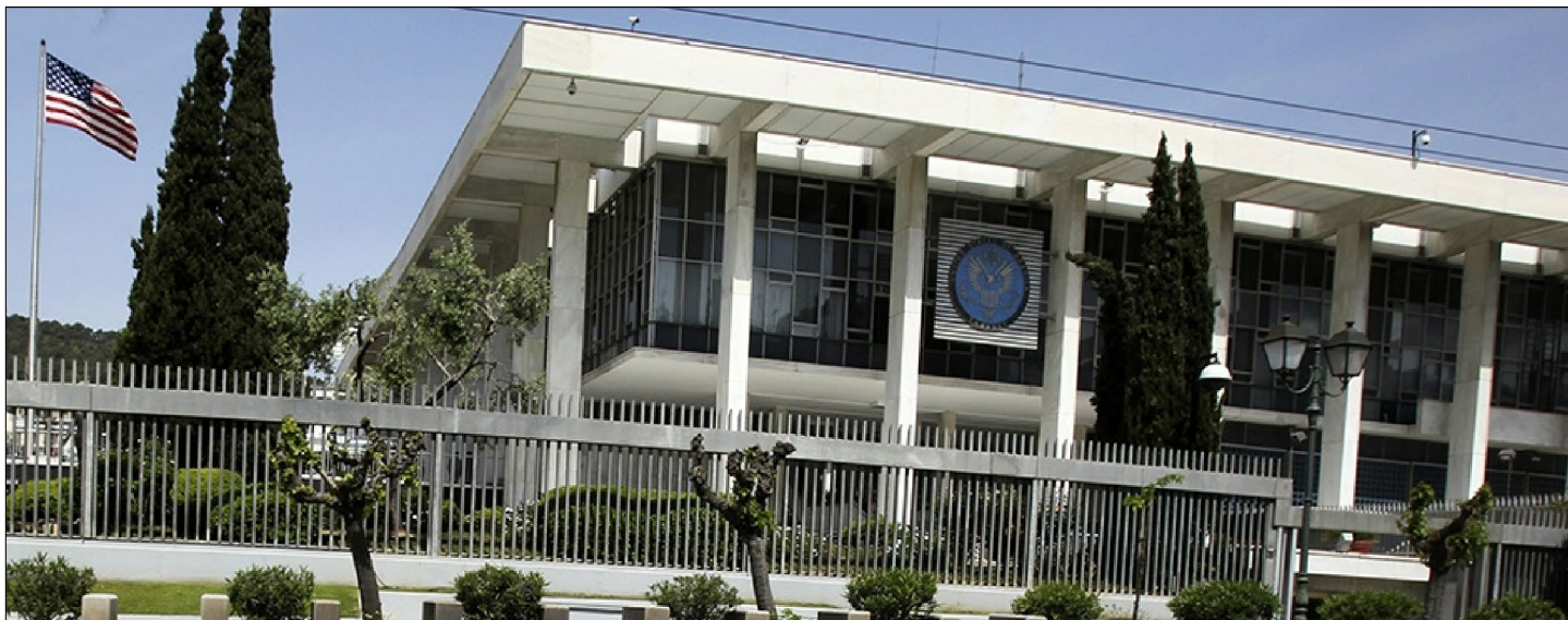
Figure 5: U.S. Embassy Athens, Greece - Example of a $343 Million, Maintenance Cost Sharing-Major Rehabilitation Project, Began in 2018 and Planned for Completion in 2023
