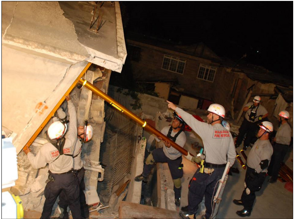
Figure 4: Example of Strut System Used by an Urban Search and Rescue Task Force
