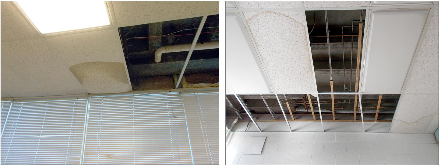
Figure 4: Damaged or Removed Classroom Ceiling Tiles Due to Leaks in Recently-Installed Roofs
