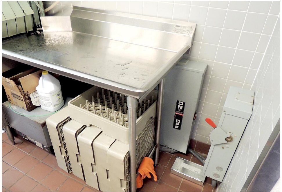
Figure 5: High Voltage Electrical Panel Installed Next to Cafeteria Dishwasher at a BIE-Operated School, October 2014
