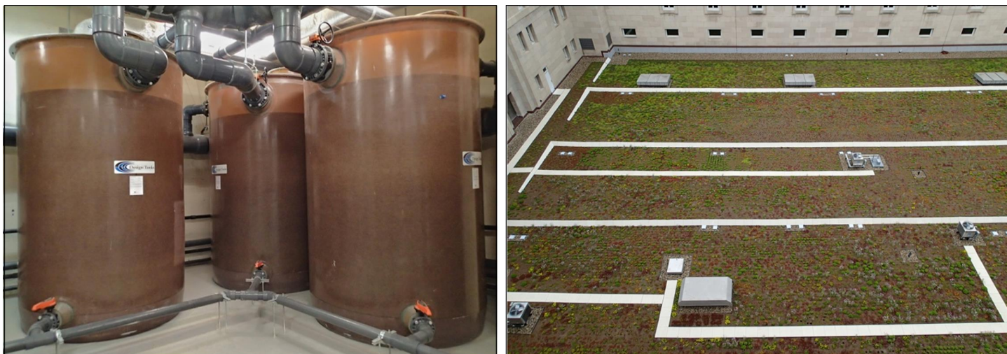
Figure 3: Storm Water Collection Tanks and Green Roof Installed at the Birch Bayh Federal Building and U.S. Courthouse in Indianapolis, Indiana
