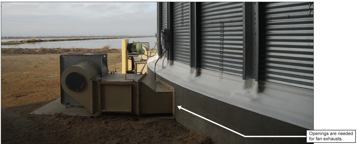
Figure 4: Rice Drying Structure, an Example of a Structure That Is Difficult to Dry Flood-proof because Openings Are Needed for Fan Exhaust (Sutter County, Calif.)
